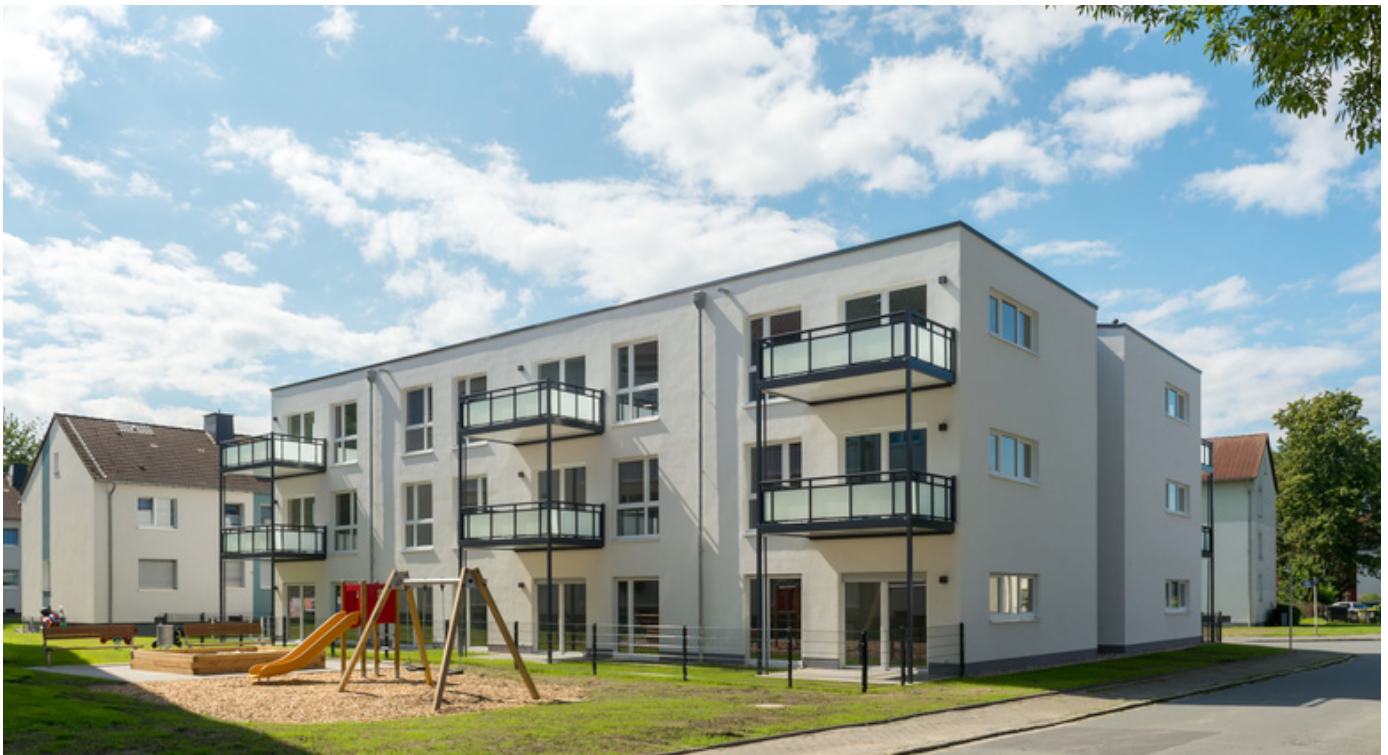
Vonovia's modular housing units in Dortmund, Brechten, Germany. Credit: Simon Bierwald, Vonovia
