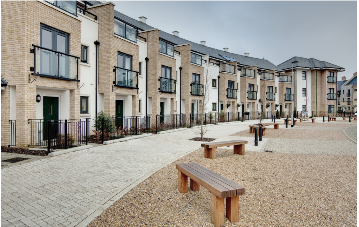
Accordia in Cambridge, United Kingdom, which includes 30 percent affordable housing. istockphoto © frazaz
